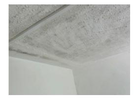
Mould growth due to condensation to ceiling to room rear left
