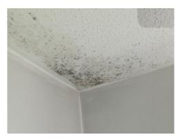
Mould growth due to condensation to ceiling to room front right
