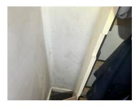
Mould growth due to condensation to walls to room front right
